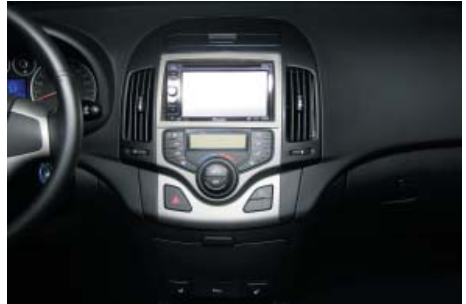
Place the back the storage bin and place the new radio trim.
